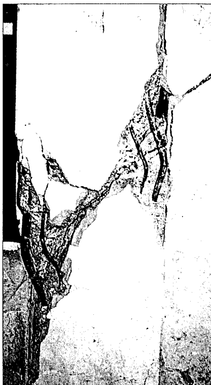
Fig. 6 — Diagonal tension failure in a column.
