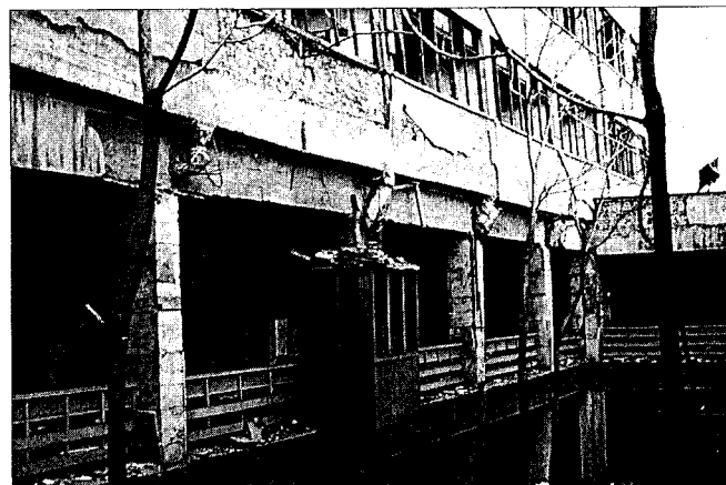
Fig. 2 — Red Crescent commercial center with strong beams and weak columns.
