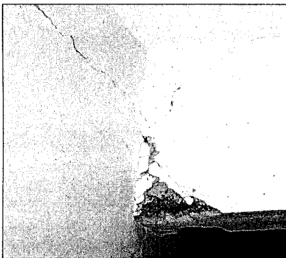
Fig. 4 — Crushing of beam cover concrete in the Officers' Club.
