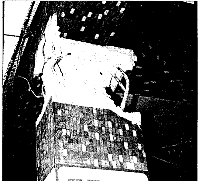
Fig. 5 — Example of lack of transverse reinforcement and resulting brittle behavior in columns.
