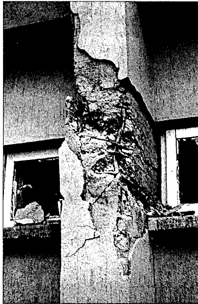
Fig. 9 — Short column behavior observed in the Police College.
