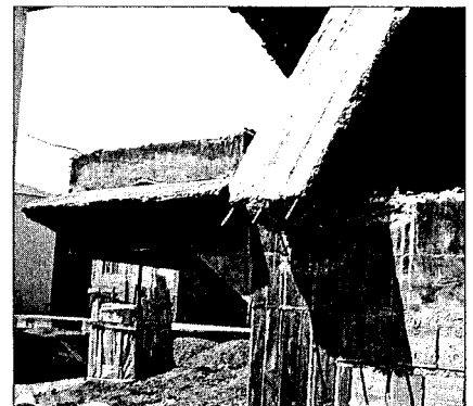
Fig. 11 — Inadequate splice length in columns.
