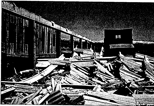
Fig. 16 — Total collapse of a precast industrial building.
