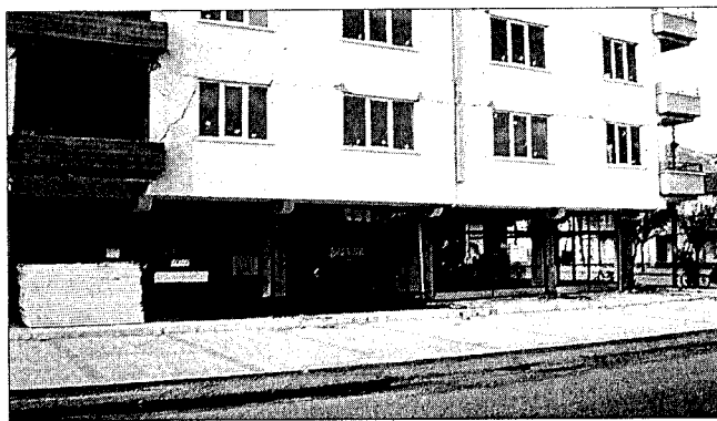
Fig. 1 — A typical apartment building with a soft story.
