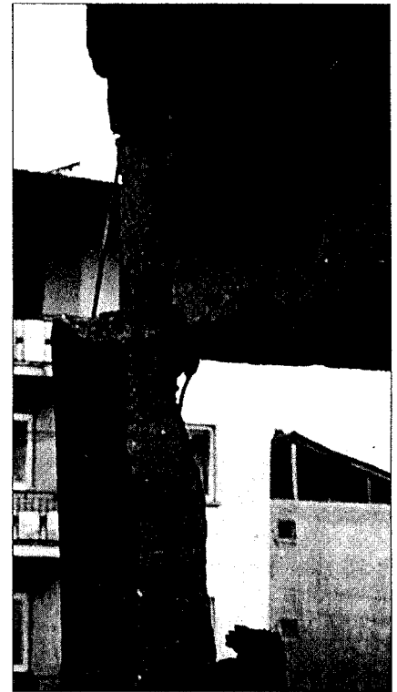
Fig. 10 — Example of poor joint detailing.
